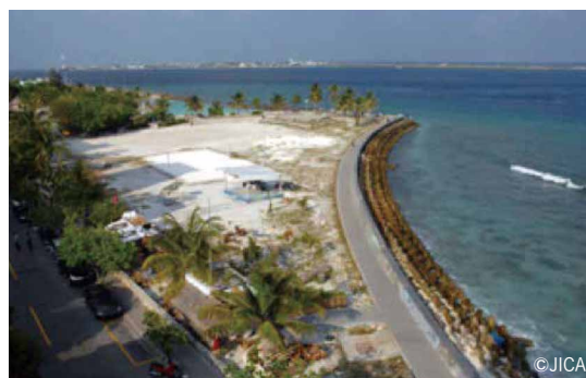
Seawalls built around the Male Island
